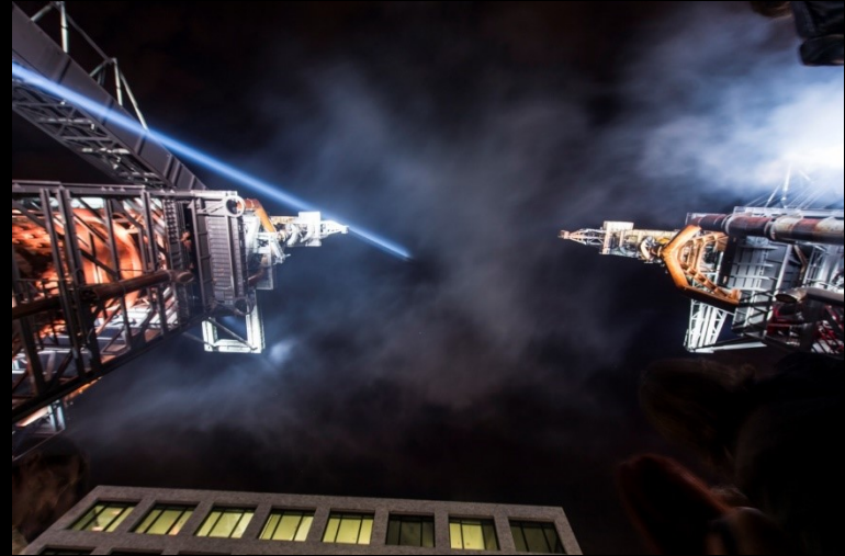
Light design blast furnaces
